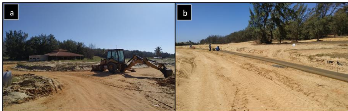
Images a and b: Construction site of Costa dos Ventos Project Source: Research archive (2021)
